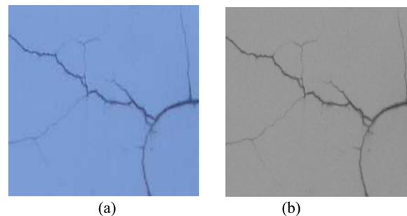
Figure 8 . Cracks that occurred on a chaotic way in an outer wall; (a)original image (b) grayscale (c) Hough
